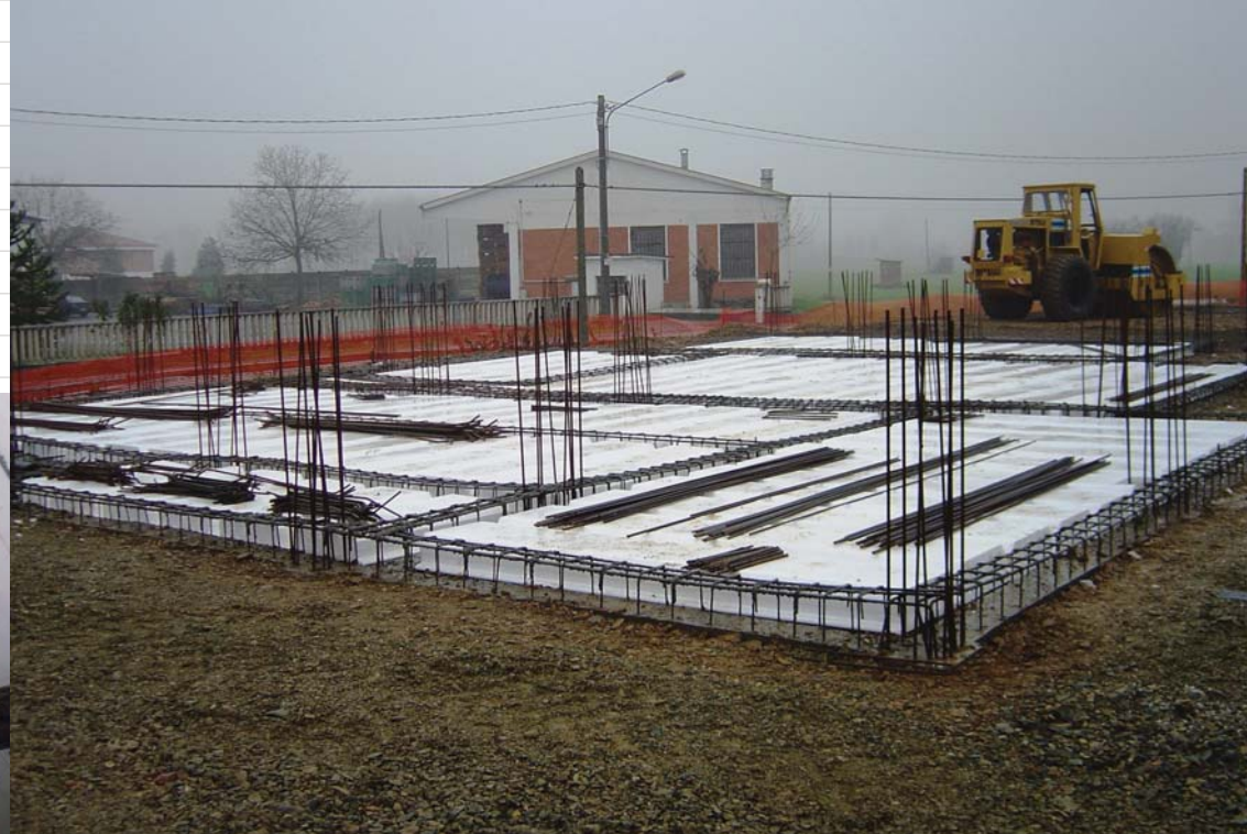
Insulated crawl space
