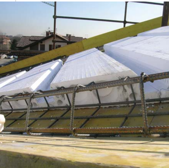
Roofing of a new building
