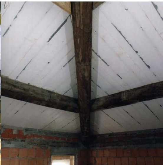
Roofing of a historic building
